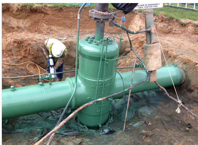
Figure 1. Spray application of an in-service 20 in. gate valve.
