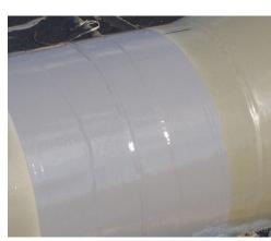
Polyclad 777 weld joint sprayed with MixCoat System
